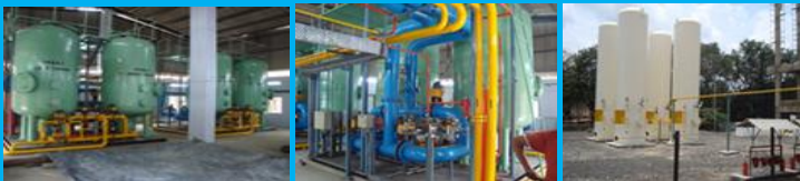
ERECTION COMMISSIONING & MAINTENANCE OF OXYGEN / NITROGEN / ACETYLENE PLANT
